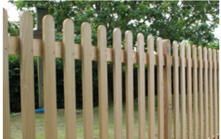
Traditional Palisade fencing is also known as picket fencing. 'Traditional' fencing is a term we use to describe a system of fencing made from vertical posts and horizontal rails, with pales fixed to the rails, supplied in kit form rather than panel form. Traditional Palisade is available with pointed or rounded pales.
