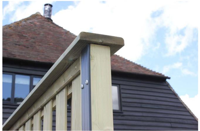
Our Mi-T post® is a modern, secure, and easy to maintain galvanised steel fence post suitable for use with our framed timber fence panels. Manufactured using high quality galvanised steel in the UK with a contemporary slimline design shaped like a 'Tee', these metal posts will not rot or rust and are guaranteed for 25 years. Their innovative design means they are not visible from the front of the fence, providing a contemporary, seamless finish in any garden.
