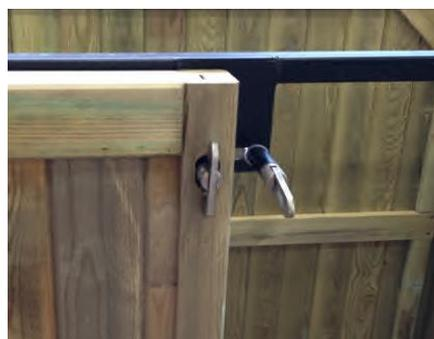
**Step 6:** Now close both doors and hold in place by latches. If the surface is flat, the top of both doors should be aligned and will have a 10-15mm gap between them (as shown below) to avoid rubbing against each other while opening and closing. If door tops are not aligned, use suitable packers e.g. washers etc. as required under a corner of the store to align them.
