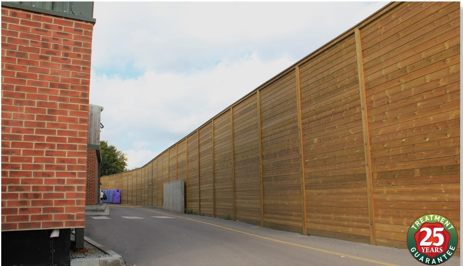
The Jakoustic® Reflective barrier is particularly effective in reflecting noise away from its face by employing heavy section planed timber boards with deep interlocking 'v' tongue and groove joints, coupled to tuning fork posts that clamp the boards together to eliminate gaps that sound could easily travel through.
