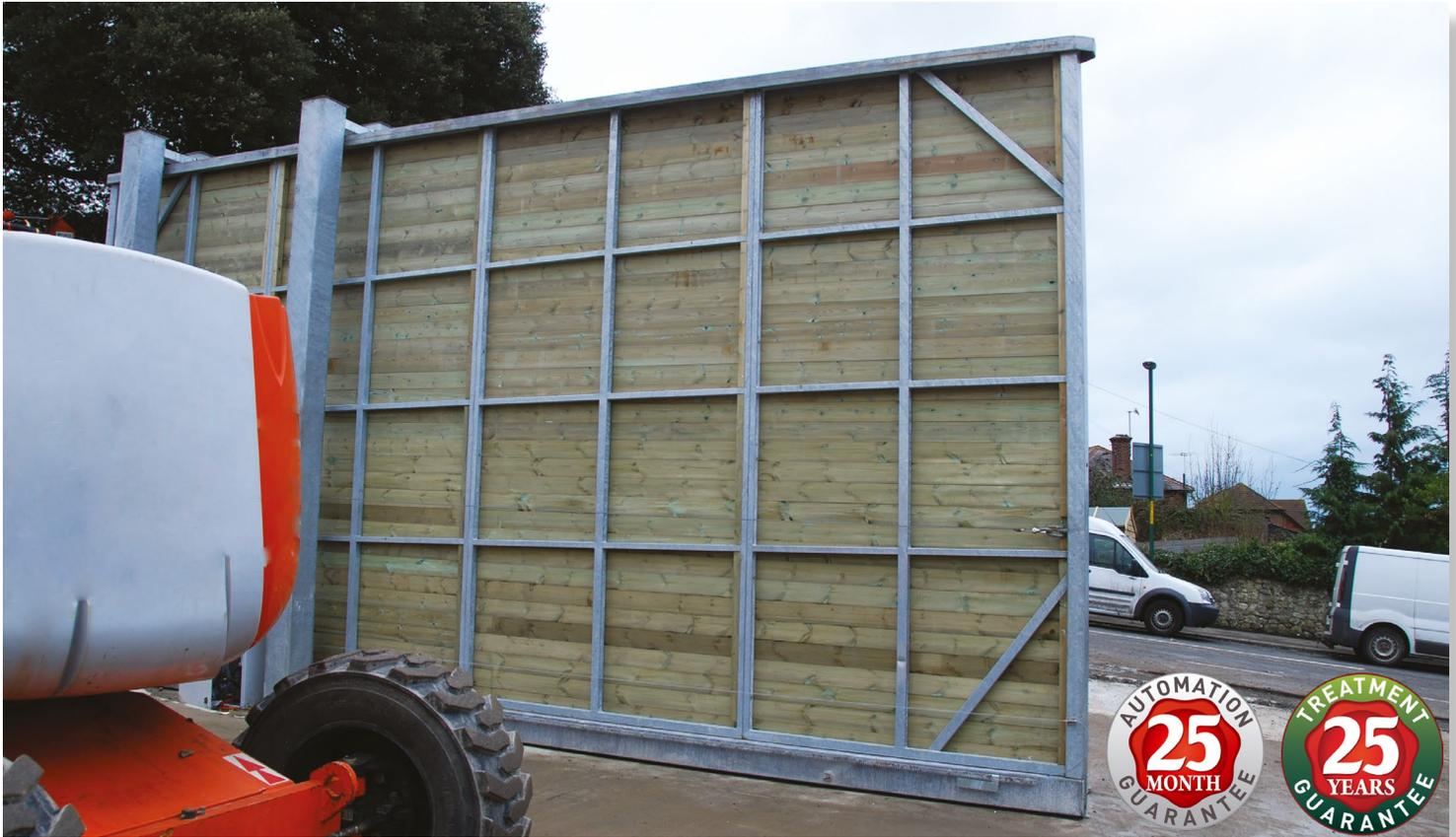
For a totally integrated, acoustic barrier solution we offer matching Jakoustic® timber or galvanised steel framed gates for pedestrian and vehicular access.
