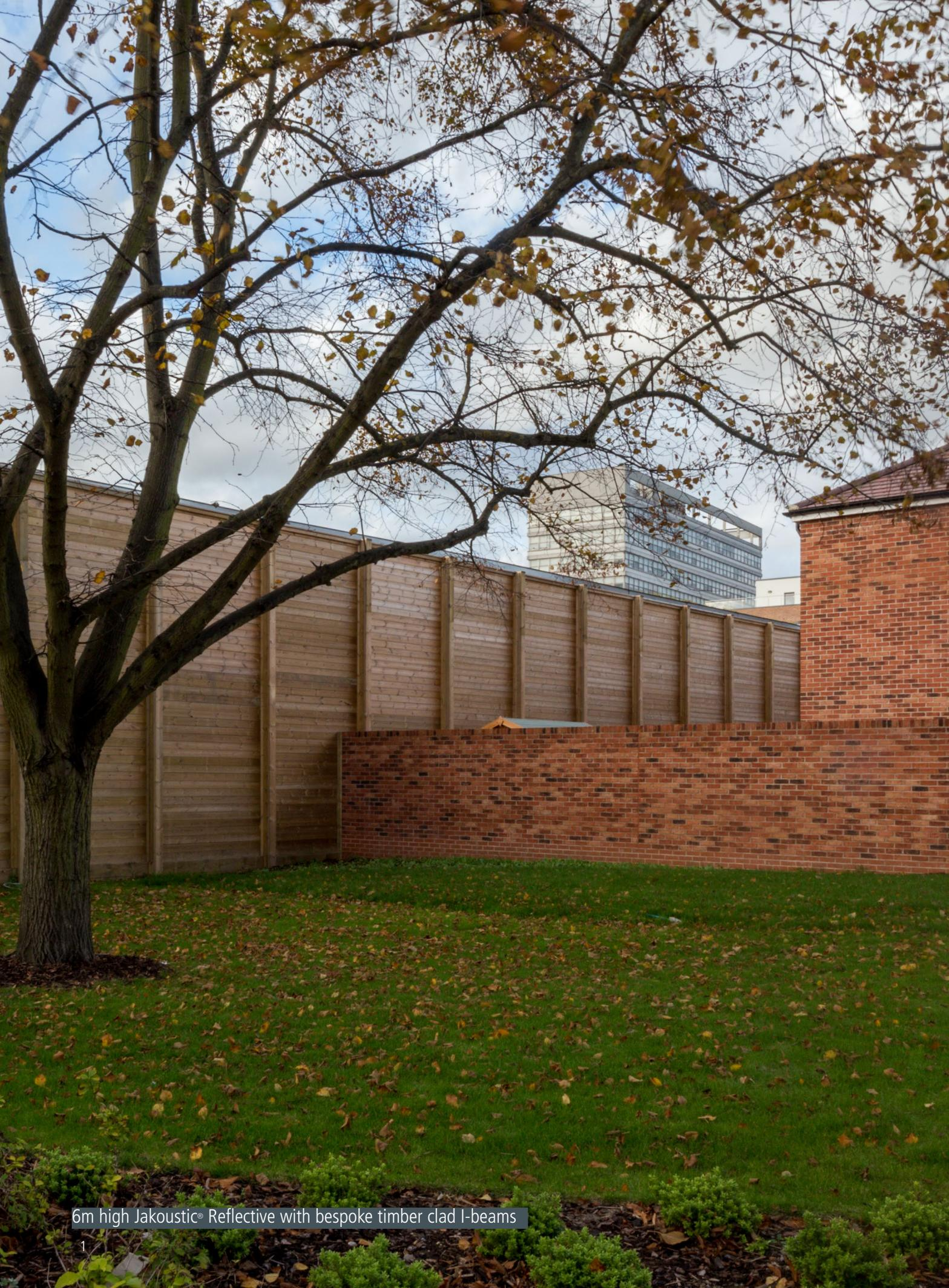
6m high Jakoustic® Reflective with bespoke timber clad I-beams
