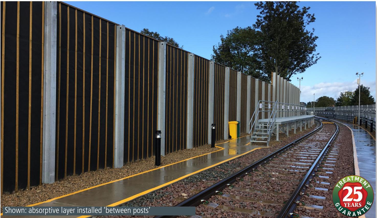
Shown: absorptive layer installed 'between posts'
