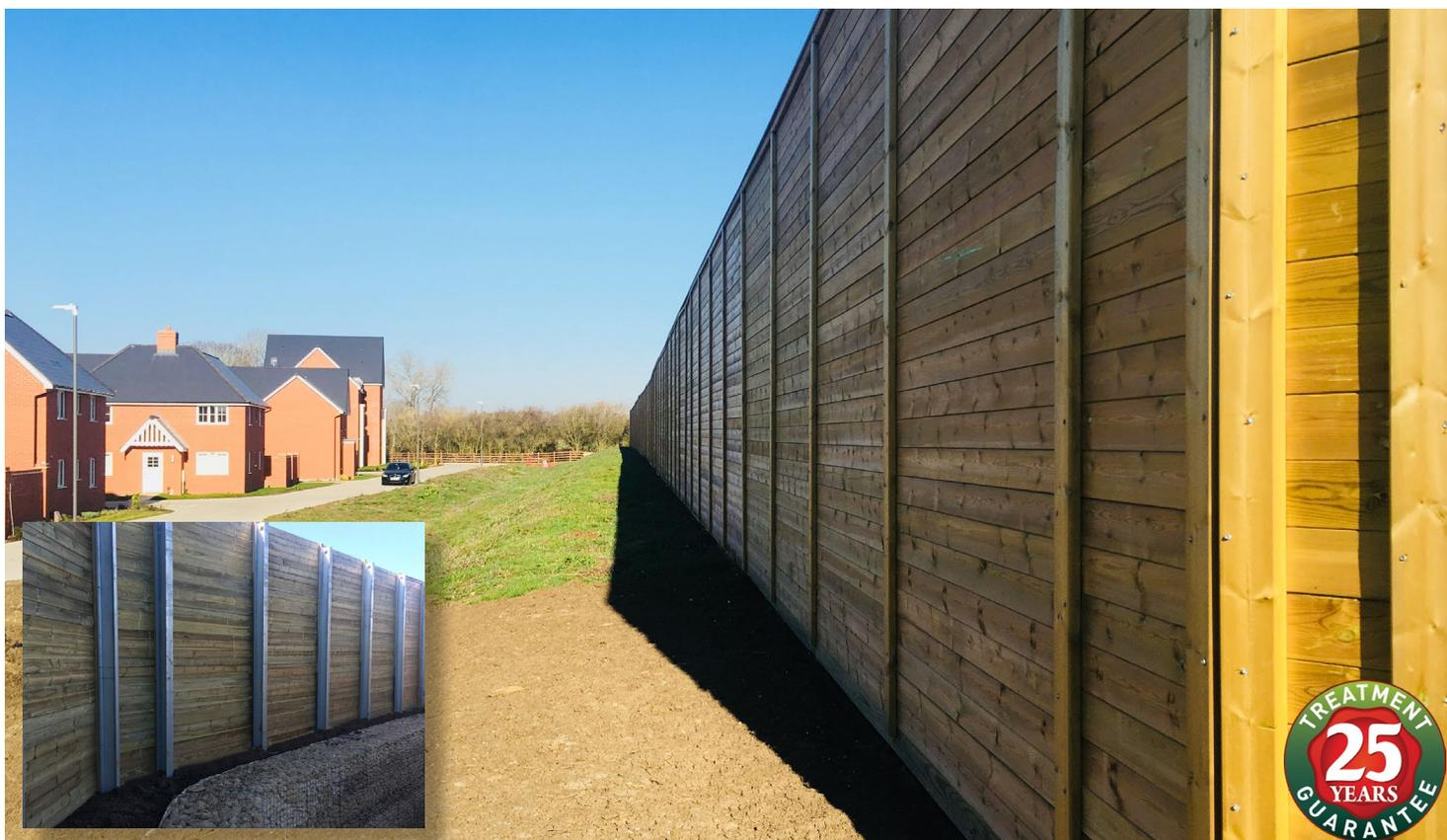
The Jakoustic® Commercial & Highway Reflective barrier system has been designed for commercial and highway applications, providing the same level of noise protection as the original Jakoustic® Reflective barrier, but it can be additionally UKCA marked as a whole system for road infrastructure.
