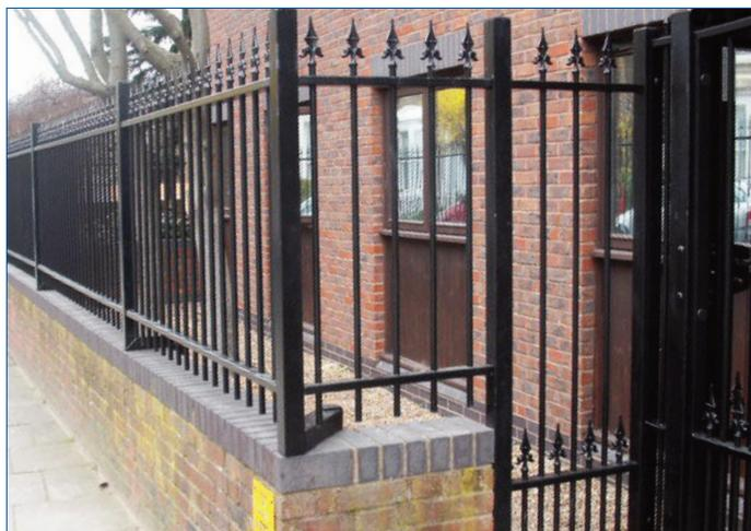
Ornamental fencing fitted with cranked posts mounted on existing wall with special width full height panel installed adjacent to the pedestrian gate
