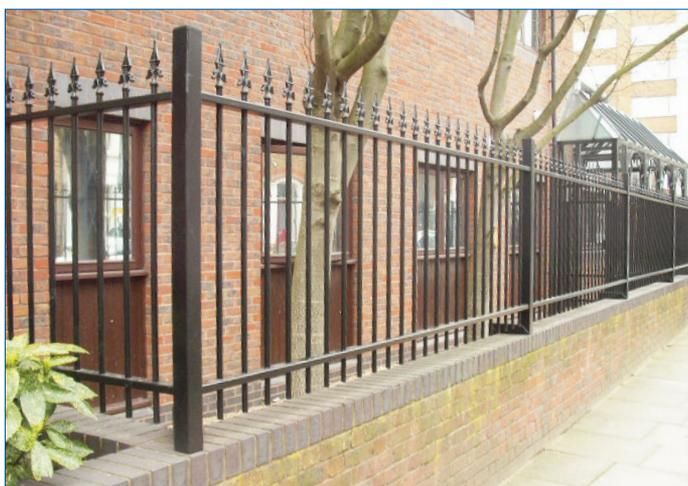
Ornamental fencing fitted with cranked posts mounted on existing wall
