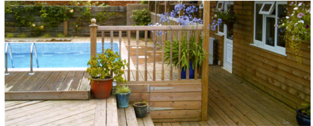
Decks are constructed with spaces between boards to aid drainage and to allow for the natural expansion and shrinkage of the timber, while all fixings and fastenings are non-rusting to ensure an extra-long life.
