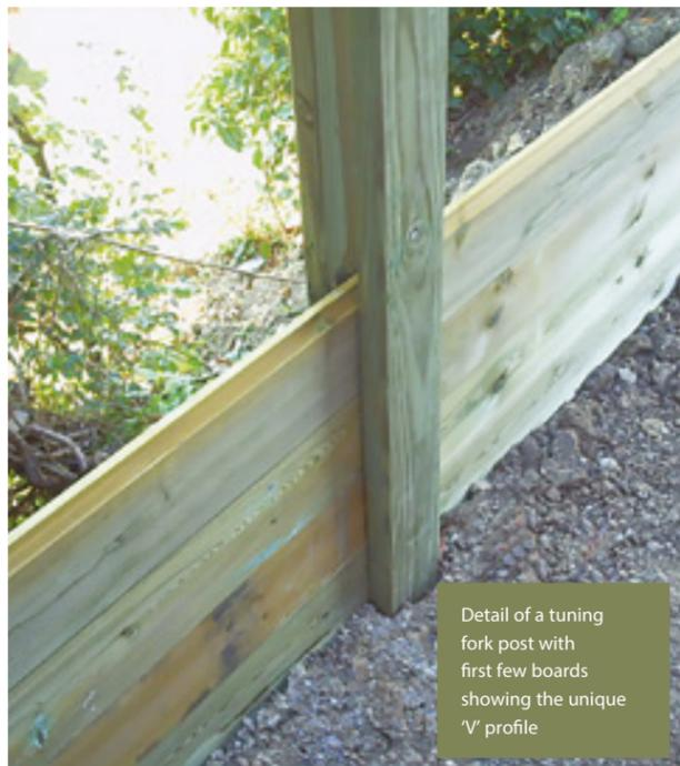
Detail of a tuning fork post with first few boards showing the unique 'V' profile
