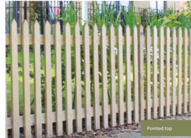
The fence should be erected 50mm above ground level to allow for weeding, and to keep it clear of the ground.
