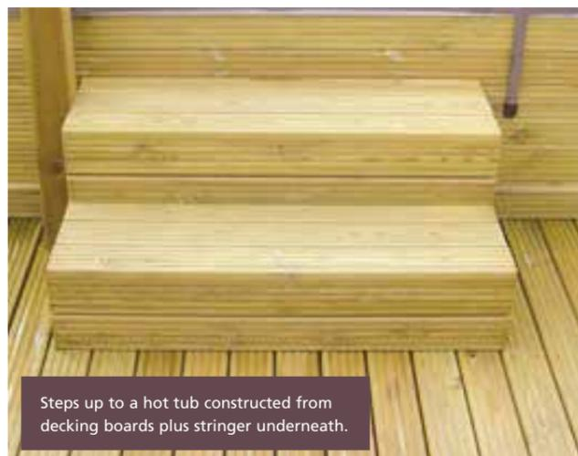
Steps up to a hot tub constructed from decking boards plus stringer underneath.
