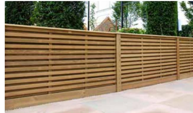
Constructed using 45mm x 16mm horizontal slats with a gap between the slats of approximately 30mm (which is larger than standard Venetian).
