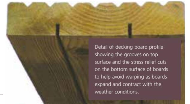
Detail of decking board profile showing the grooves on top surface and the stress relief cuts on the bottom surface of boards to help avoid warping as boards expand and contract with the weather conditions.
