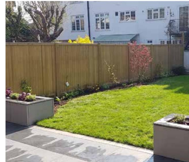
The centre of the panel is given additional support with one 70mm wide rail for heights up to 1.22m, and two rails for heights of 1.52m and above. Panels are 1.83m wide, available in five heights from 0.91m to 1.83m with the option to use a panel width cut-down kit if required. Top and bottom rails are 70mm x 51mm planed with sides of 45mm x 51mm. Standard Tongue and Groove Effect panels have 21 pales.
