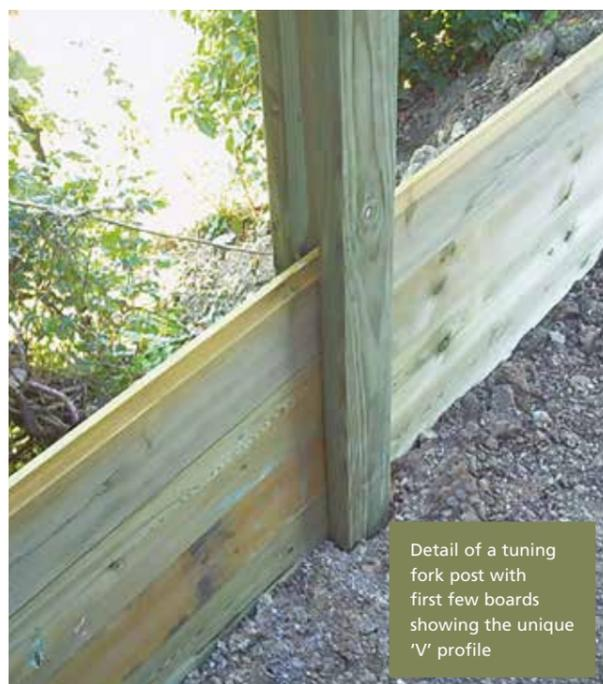
Detail of a tuning fork post with first few boards showing the unique 'V' profile
