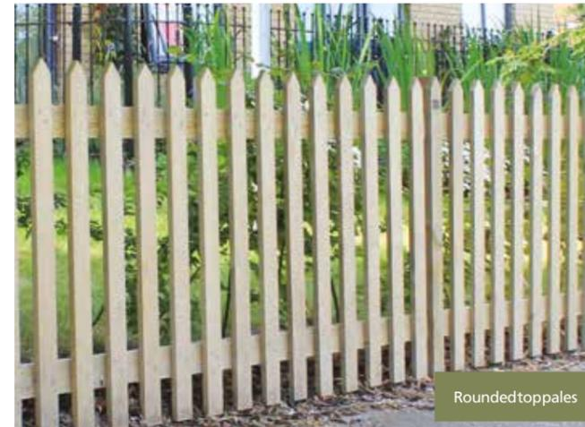
The fence should be erected 50mm above ground level to allow for weeding, and to keep it clear of the ground.
