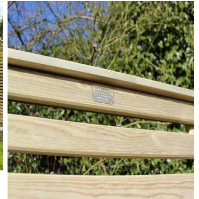
The key difference is that the fence posts are less visible, meaning that, when installed, the panel will appear as continuous slats, rather than a run of individual panels.
