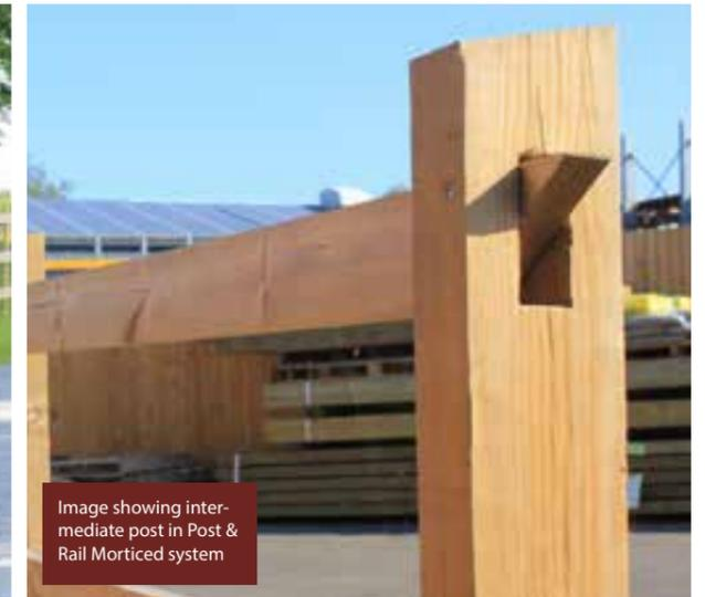
Allow one post and one prick post for every 2.85m of fence, plus one post for the end of the run. Allow three rails per 2.85m run of 3-rail fence, and four rails per 2.85m of 4-rail fence.
